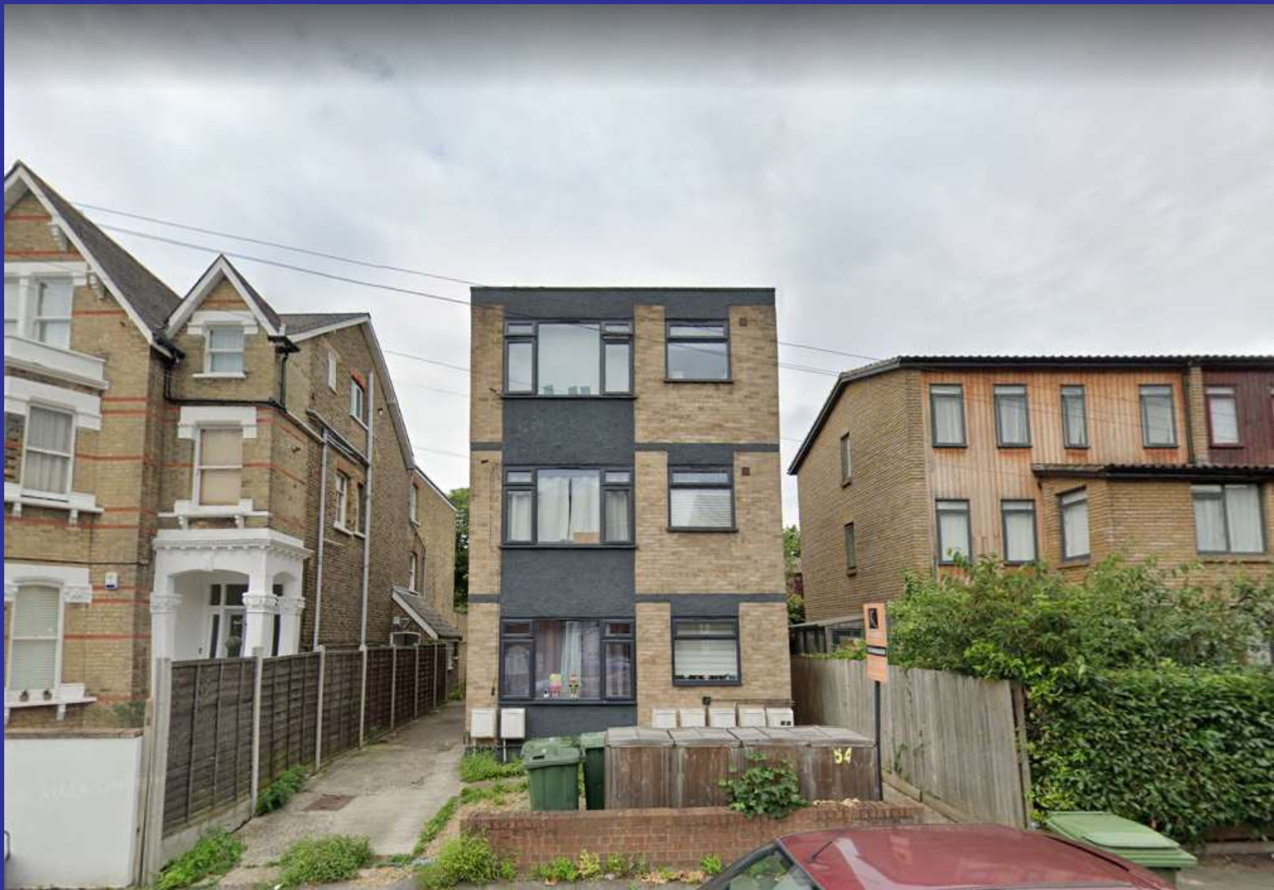
Existing three storey property
